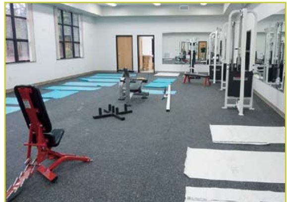
Workout room at new Mukwa Health and Fitness Education Center begins to take shape.
