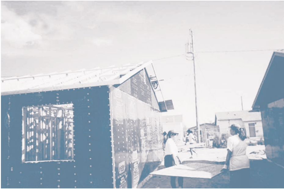
The Mercy Loan Fund has worked with the Housing Assistance Council to fund Arena Dorado, a self-help homeownership program for farmworker families in the colonias near Anthony, New Mexico.
