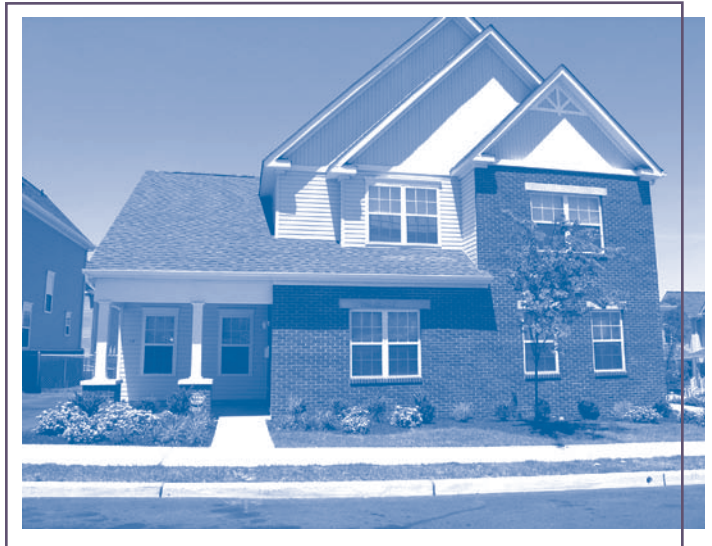
Baldwin's Run in Camden, NJ uses HUD HOPE VI funding to reinvigorate the community through attractive, affordable housing.
