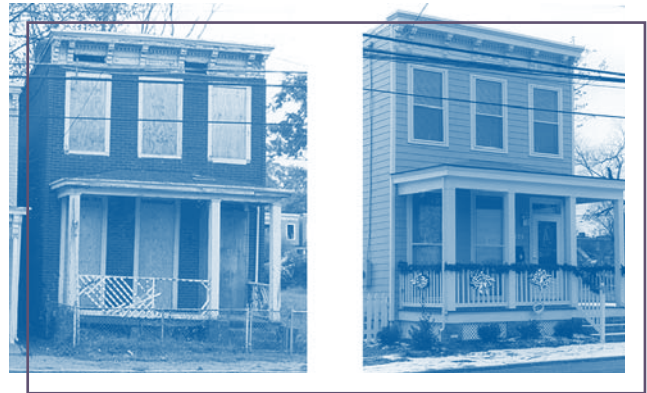
Before and after photos of a house in Carver-Newtonne West demonstrate how Richmond's Neighborhoods in Bloom program is attracting residents back into urban neighborhoods.
