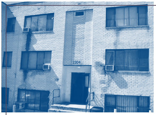
This deteriorating building was reduced to walls and studs during renovation.
