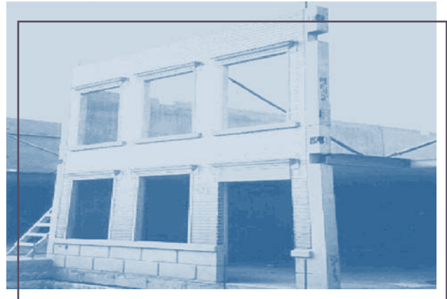
Panelized construction reduces the time required to erect a building and provides energy savings.
