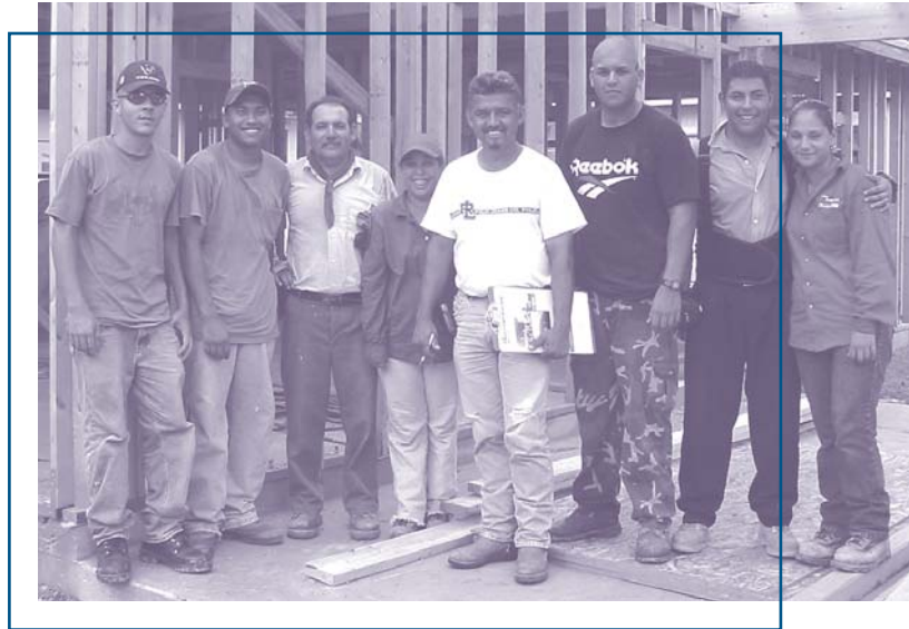
The crew that erected the framing on the PATH demonstration home in Cameron Park takes time out to pose for a picture.
