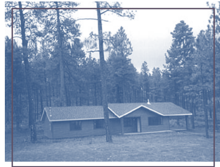
A home on the White Mountain Apache reservation made possible with a Section 184 loan guarantee.
