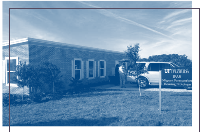
The Migrant Worker Prototype House was constructed and finished in five weeks.
