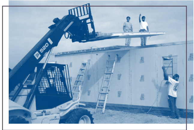
Installation of SIPs requires fewer construction workers than traditional construction methods.
