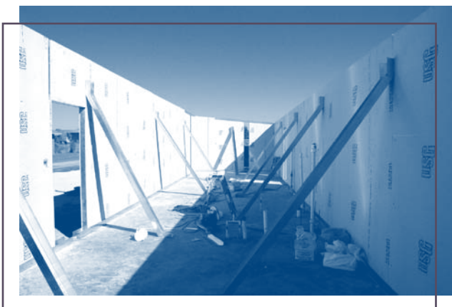
Structural insulated panels (SIPs) are energy-efficient, mold- and mildew-resistant, and can withstand Category 4 hurricane winds.
