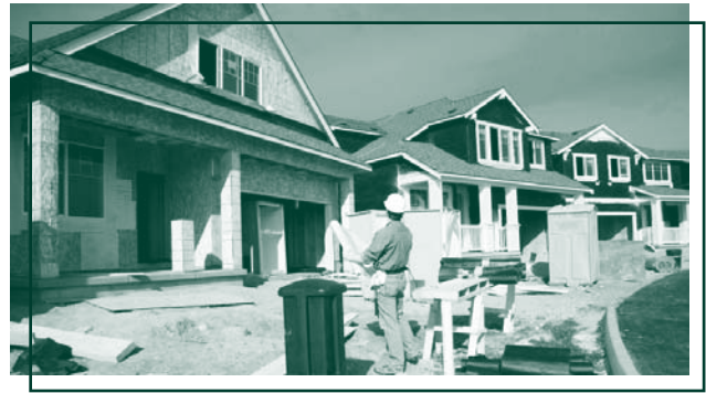
Site-built, or stick-built, housing is constructed entirely on location.
