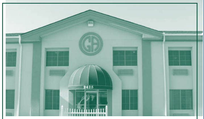
Gosnold Apartments provide affordable housing for 60 formerly homeless individuals from Norfolk, Virginia Beach, and Portsmouth. The former bottling plant is the nation's first regional housing project.
