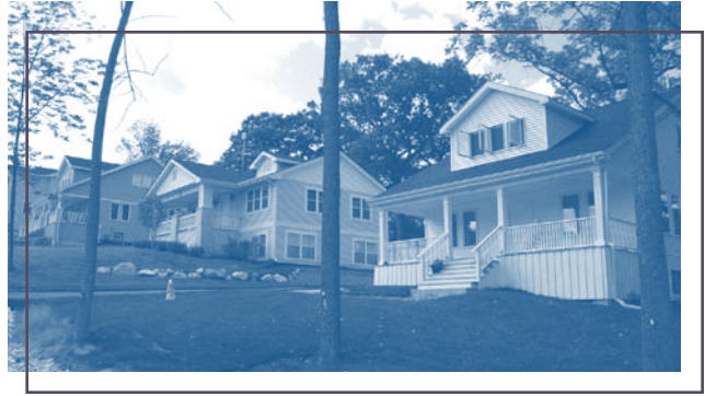
The five Owasco Avenue houses resemble the traditional bungalow-style homes commonly found in Elgin neighborhoods.
