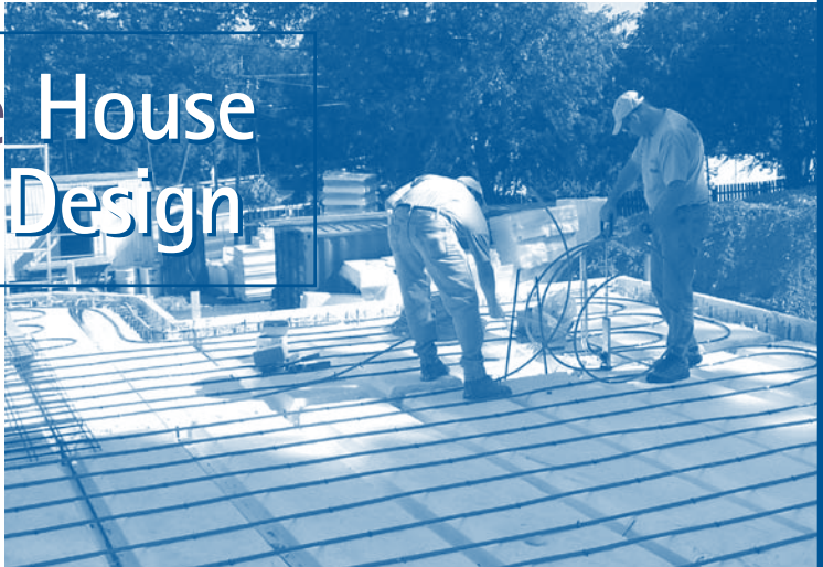
Workers connect a radiant floor heating system in the Paterson Showhouse.
